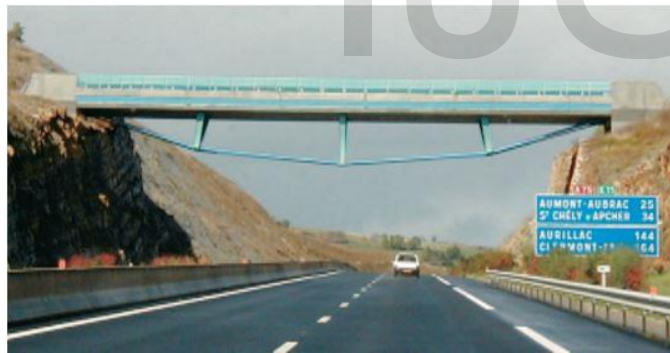
Figure 1-1 Truc de la Fare overpass, France 1993, Simply supported span road bridge with a span of 53m, prestressed concrete deck with 8m width, span to depth ratio 1/33 [1].
